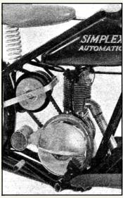
"free-engine" position and, afterwards, automatically raising or lowering the gear according to throttle opening and gradient. Thus, driving consists solely of operating the twistgrip and the brake pedal—the acme of simplicity.
