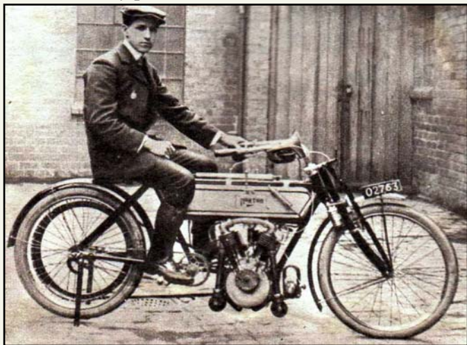
Rem Fowler aboard his 1907 twin. This picture was taken in a hurry as the magneto has been mounted back to front. This machine made the fastest lap of the first TT in 1907 and won the twin class.
